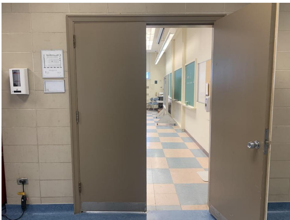
Image Description: The doors entering the room have a doorknob on the left hand side and are not opened by an automatic door controller.
