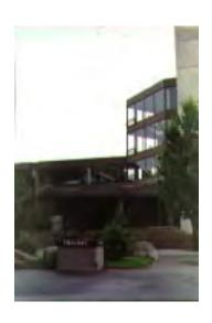
The main building has 4 storey sections flanking a central skylit internal pedestrian "street". The exterior walls are of poured concrete with deeply recessed horizontal windows under a flat roof. The interior walkway consists of vinyl composite flooring, painted drywall, and untreated concrete columns.
