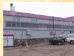
Solar panels on the Nunavut Arctic College
