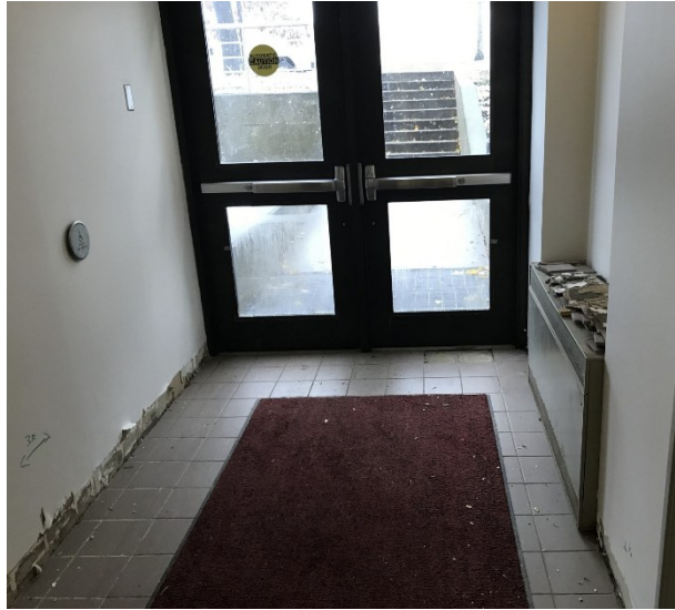
Figure 2: Water Damage to Sutherland Hall in 2019 (Queens Facilities 2024)
