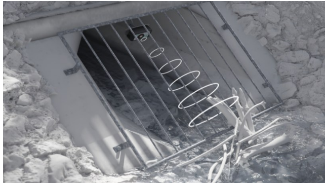
Figure 18: IOT Ultrasonic Sensor installed inside Grate (“Reliable Remote Monitoring of Drain Grates” 2024)
