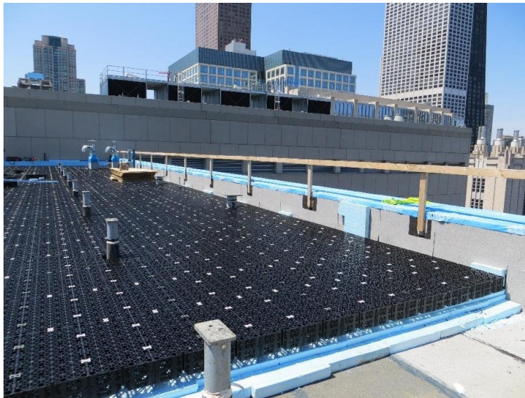
Figure 5: Example of Blue-Roof System (“Unlocking Stormwater Solutions: A Northwestern University Case Study on Blue and Green Roofs” 2023)
