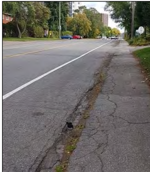
Figure B-17: Broken asphalt on paved shoulder of Richmond Road.
