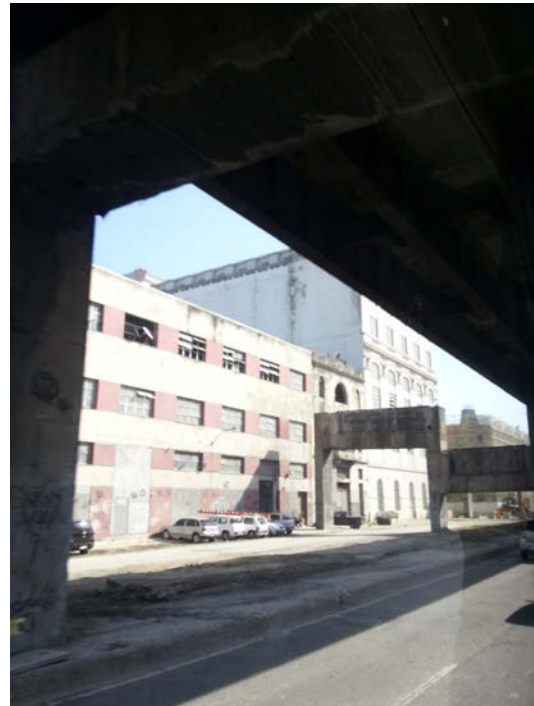
Figure 3 Federal and State capital are funding the removal and replacement of an elevated expressway with an LRT in Port Maravilha
