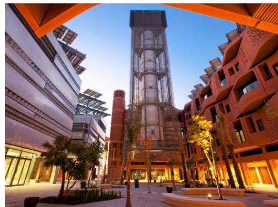
At one of the public square is a contemporary re-interpretation of the traditional Arabic wind tower, which has been designed to bring cooling breezes down to ground level.
