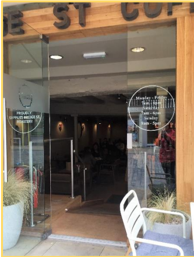
At level and ramp access at a cafe
