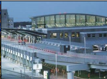
Warwick Station, Rhode Island
