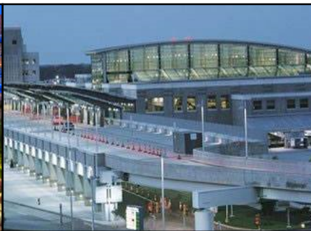
Warwick Station, Rhode Island
