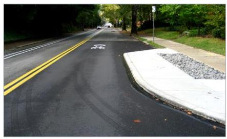
**Figure 7.7:** Example of a curb extension and a sharrow in Squirrel Hill, Pittsburgh (Bike Pittsburgh, 2009).
