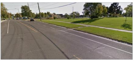
**Figure 4.14**: Portsmouth Avenue, facing south towards King Street. The bike lane on the right abruptly ends and becomes a right turn channel for motorists. This poses a challenge for cyclists attempting to travel south (Newton, 2014).
