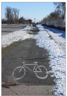
Figure 5.2: One of Kingston's few separated cycling lanes (east of Lake Ontario Park, south of King Street), along a key route to access the hospital, is left unusable due to snow buildup (Newton, 2014).
