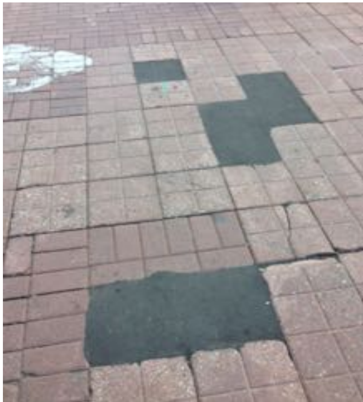
Asphalt patches and brick repairs along the Sparks Street Right-of-Way.
