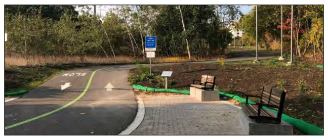
Image 94: Mixed asphalt and permeable pavement pathway with seating along the Lower Don Pathway.
