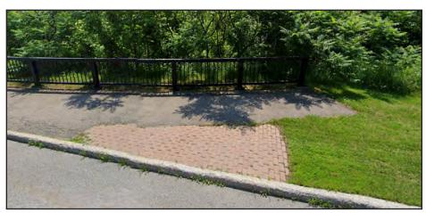
Image 49: Abrupt beginning of pathway on SGEC Parkway (eastbound) at Green's Creek Overpass. There is no crossing for pedestrians to safely access this from the Ottawa River Pathway, and the curb is not dropped for cyclists, strollers or wheelchairs to access (Google, 2019a).
