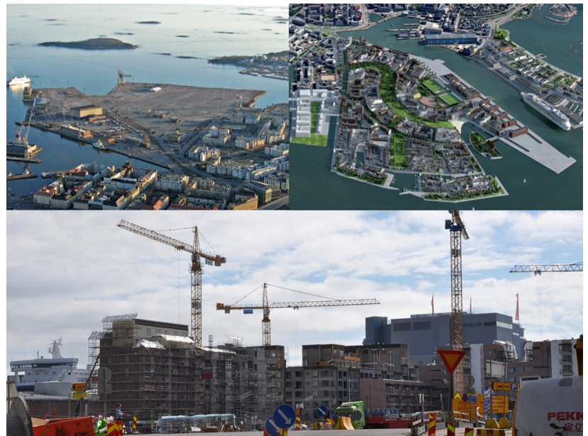
Figure 3. Jatkaasari is just one of Helsinki's former port land areas being redeveloped as an urban neighbourhood. As you can see, construction is well underway.
