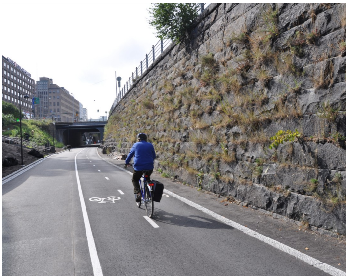
Former off-ramp recently transformed into a segregated bikeway.
