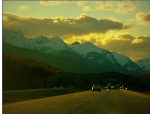
Wildlife overpass, Trans-Canada Hwy, Banff, AB. Credit: Anita Sott, 2012.
