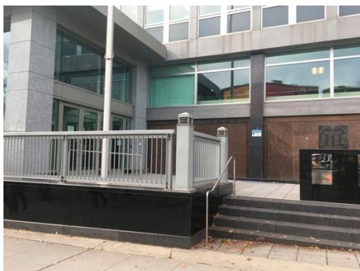
Figure 4: British High Commission security retrofit
