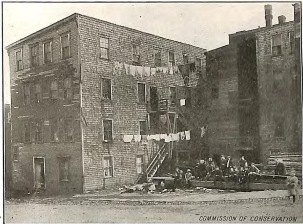
Four storey tenement house in a Canadian city occupied by eight families.
