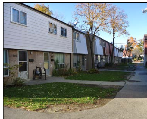
Figure 1: Townhouse units in Chester Le
