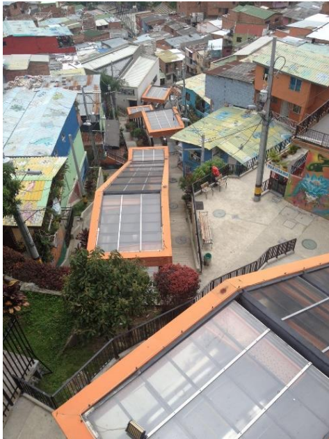
Escalators wind up the hillside of an informal settlement helping to integrate the neighbourhood through increased accessibility.
