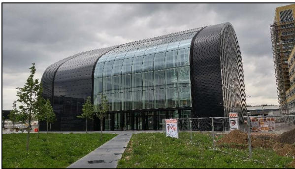
Bruxelles Environnement’s new building in the Docklands neighbourhood is the second-largest passive energy building in Europe, and the largest in Belgium.
