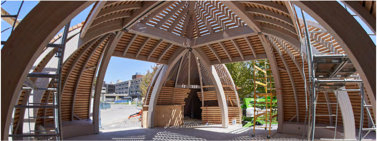
Construction progress on the new Indigenous Gathering Space.
