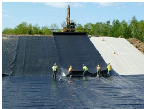
Fig 1 Dr. Kerry Rowe and his team install a liner at the Queen's University Environmental Liner Test Site in Godfrey, Ontario
