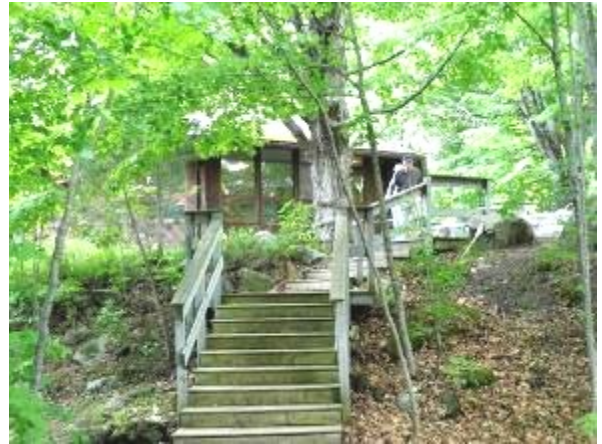
Elbow Lake Biology Station Club House
