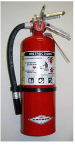
5. Visually inspect the extinguishers for dents, leaks, rust, chemical deposits or other signs of abuse/wear. If an extinguisher is damaged report this information the Department of Environmental Health & Safety (32999).
