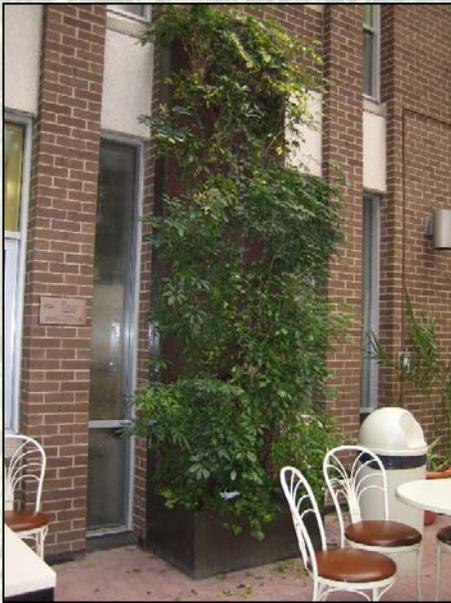
**Figure 5: A Passive Biowall at the University of Waterloo**
