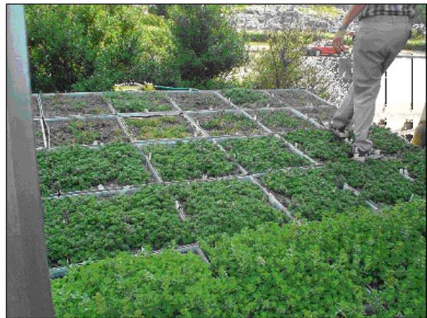
**Figure 3. Modular green roof systems<sup>14</sup>**
